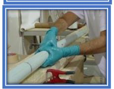
(See building notes for complete text) Pull the sleeve as tight as possible: And apply resin
