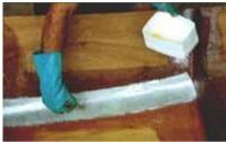
The resin will cure (harden) and the result, seam or panel, will be a strong, hard fiberglass part. That is all! **Epoxy & Fiberglass basics**
