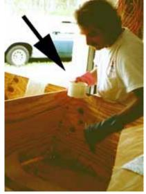
We need some putty to fill the corner first. The putty is made very easily from resin mixed with a filler: micro-balloons, <u>wood flour</u> etc. It can be applied with a spatula but we describe better methods in our "Stitch and Glue" manual. Note that all surfaces are pre-coated before the application of putty or fiberglass.
