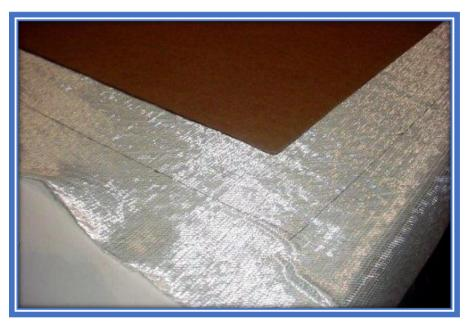
The <u>1708</u> is cut to fit and laminated into the "mold". Layers overlap 4" progressively. First layer goes 4" up sides and bottom, second goes up 8".
