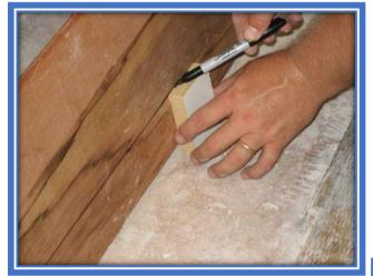
The hull is on a cradle. The purpose of the cradle is to make sure the hull is straight before glassing in the new stringers. The new stringers are made, they will go in the boat next week. Once they are
