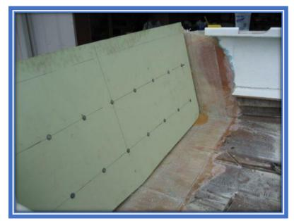
We rolled a coat of unthickened epoxy onto the core and the inside skin before the glue was applied with the notched spreader. Glue was applied to both the core and the skin. The core was "hung" on the skin. Bolts were tightened beginning with the inside and working out. Any material squeezed out was removed.
