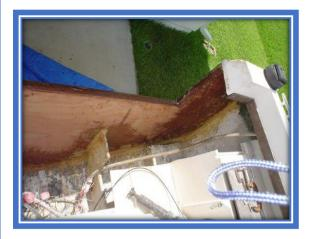
After 3 layers total, we have the total core thickness epoxied into place.
