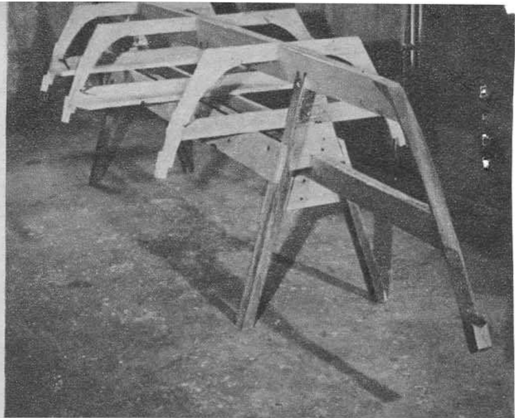
STEM, FRAMES, transom set up on building jig. Make sure 2 by 6-in. plank is well dried.
