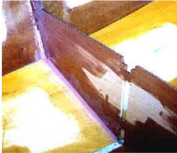
Lay the fiberglass tape on the wet putty.
