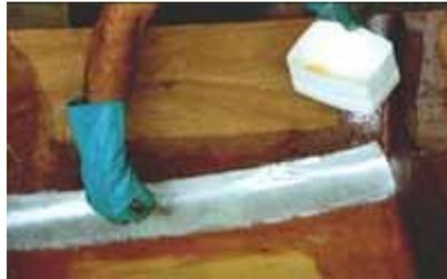
Use a squeegee to remove the excess resin and eliminate air bubbles.
