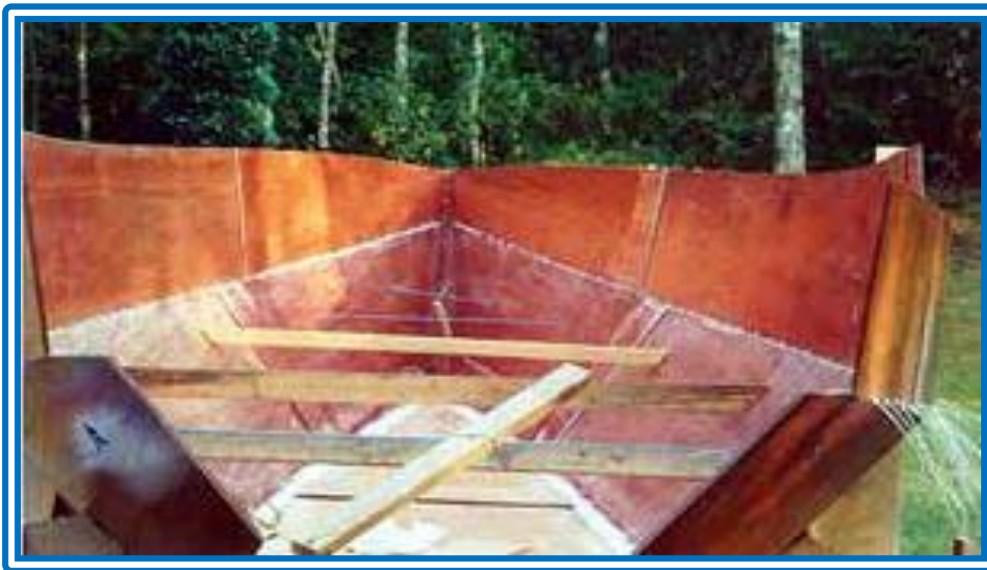
Note the spreaders that keep the panels in the proper shape
